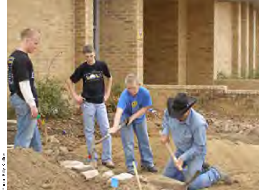
Community volunteers (left to right) Trevor Brawley, Garrett Murff, Aaron Brawley and Shawn Murff shape soil to create swales/depressions to capture rainwater for deep-rooted native plants.
